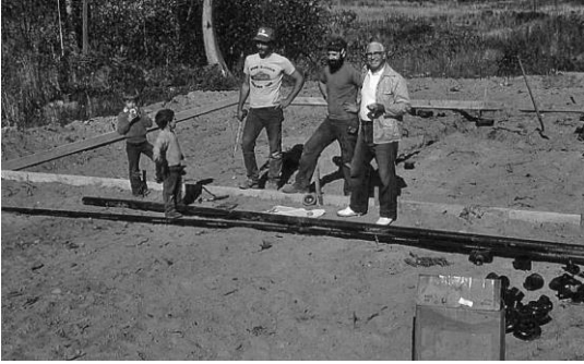
Scott Lincoln & Steve Carter donated their time plumbing the restroom building.
