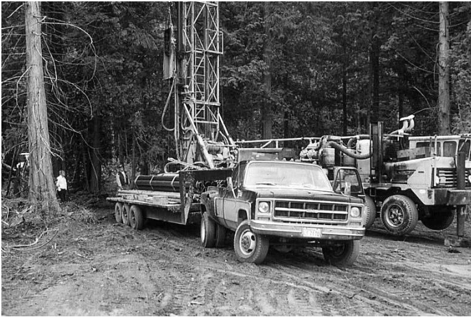
Joe Lehman drilling the well.
