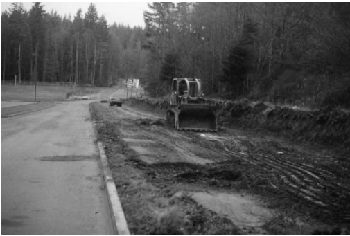
Excavating the Gabelein easement.
