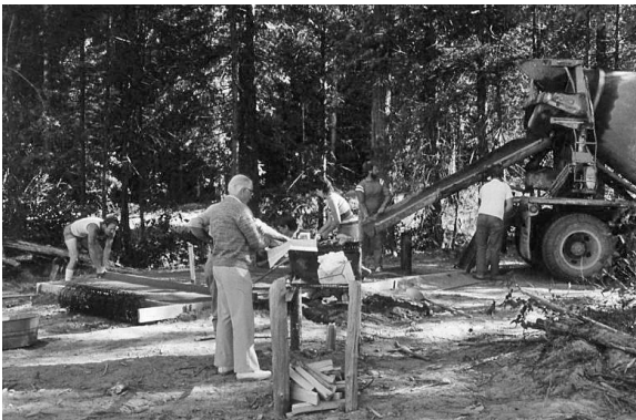
Pouring concrete for the well house floor.
