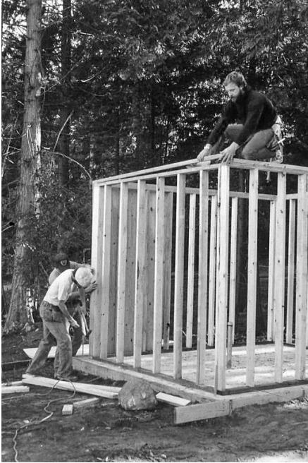
Dave Johnson, Tom Permenter and Chris Hershey framing the well house.
