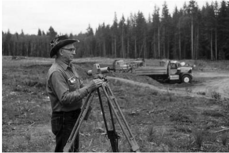
Hanford Thayer- surveying for the excavation of the south athletic field.
