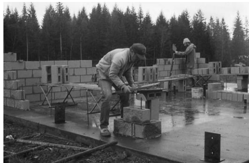
Jim Odle and Tom Permenter laying cement blocks.
