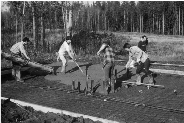
Ken Bloom, Todd Dubach and Mark Myres pouring the concrete floor.
