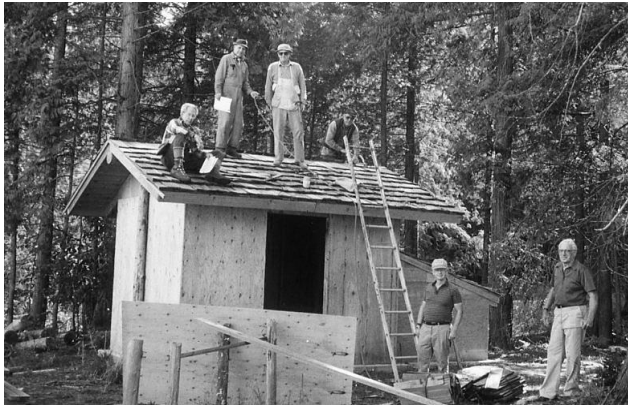
Lions Club members putting the shakes on the well house. The shakes were purchased by the Kiwanis Club.
