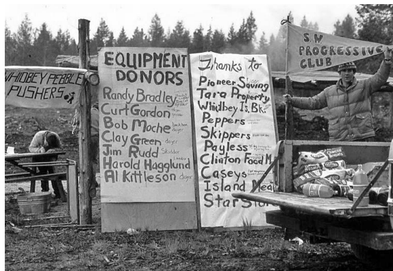
Donors who contributed to the success of one of the first work parties where heavy equipment was used.
